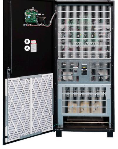
FIGURE 5.6 – 80-100KVA CABINET EXTERNAL WARNING LABEL LOCATIONS
